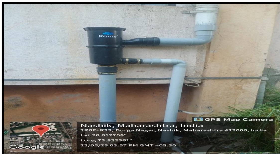
Rain water harvesting facility
